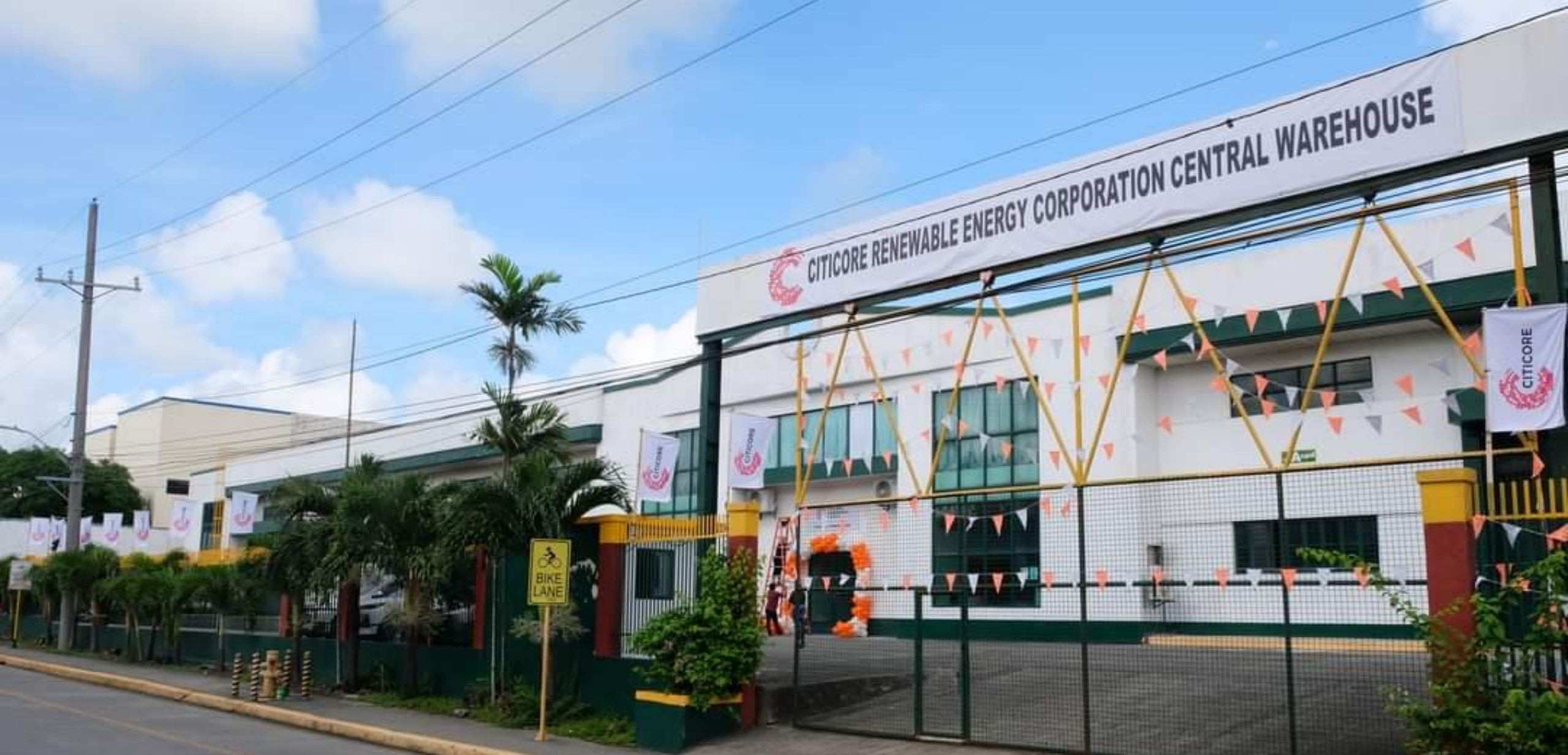
CREC Central Warehouse Inauguration | 09 June 2023
