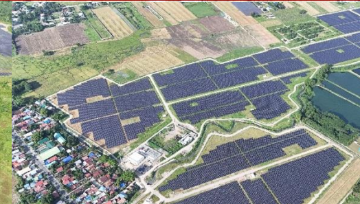
Arayat 3A – 42.0 MWp
